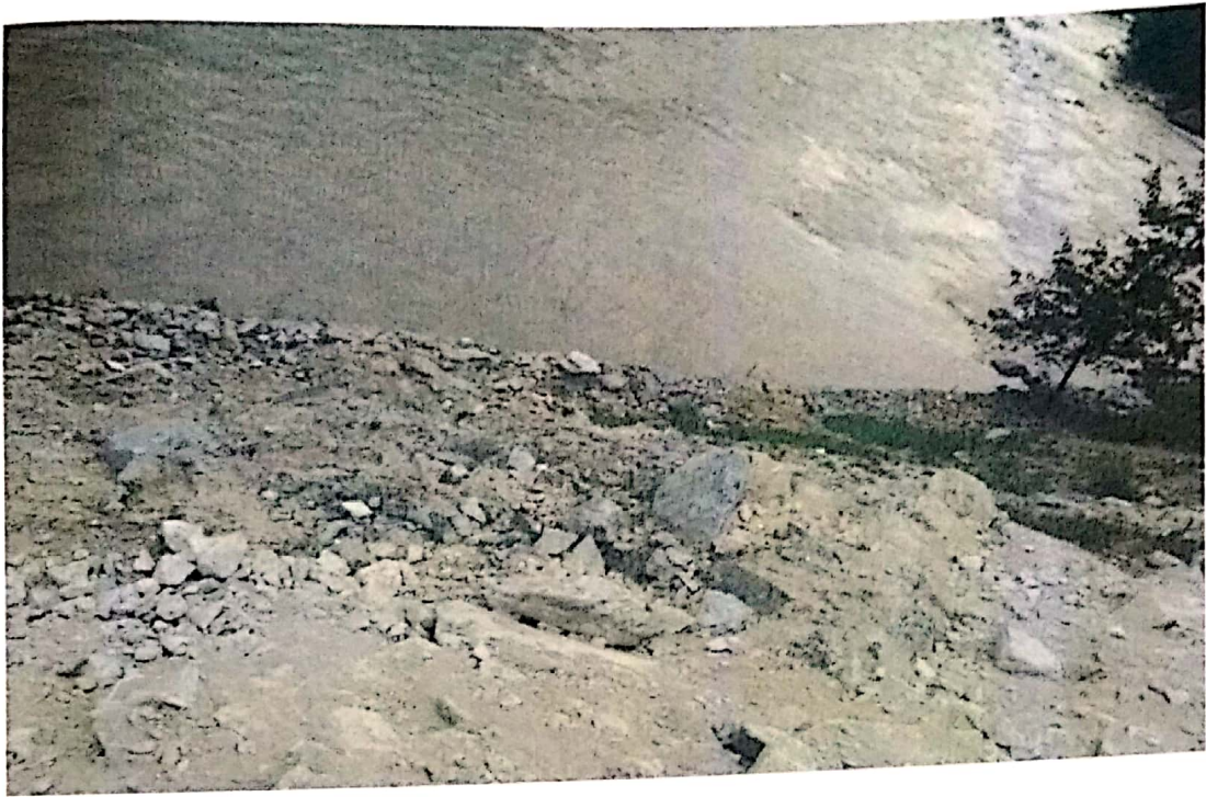
7. Muck dumped and protected adjoining river Beas: East side.
