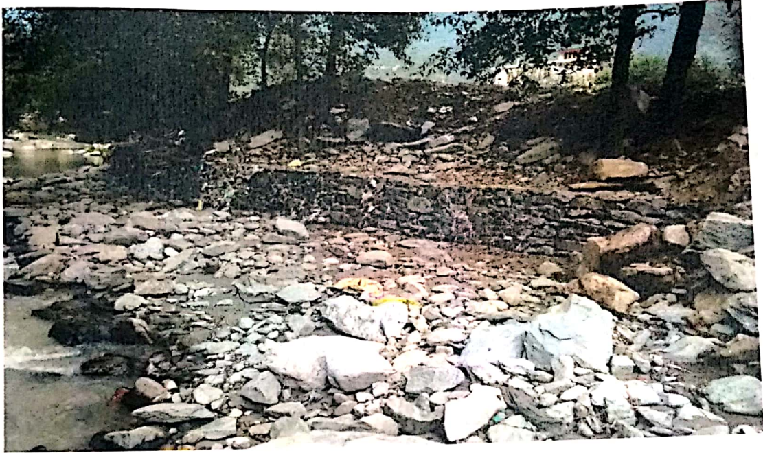
5. Muck dumped and protetced towards river Beas.
