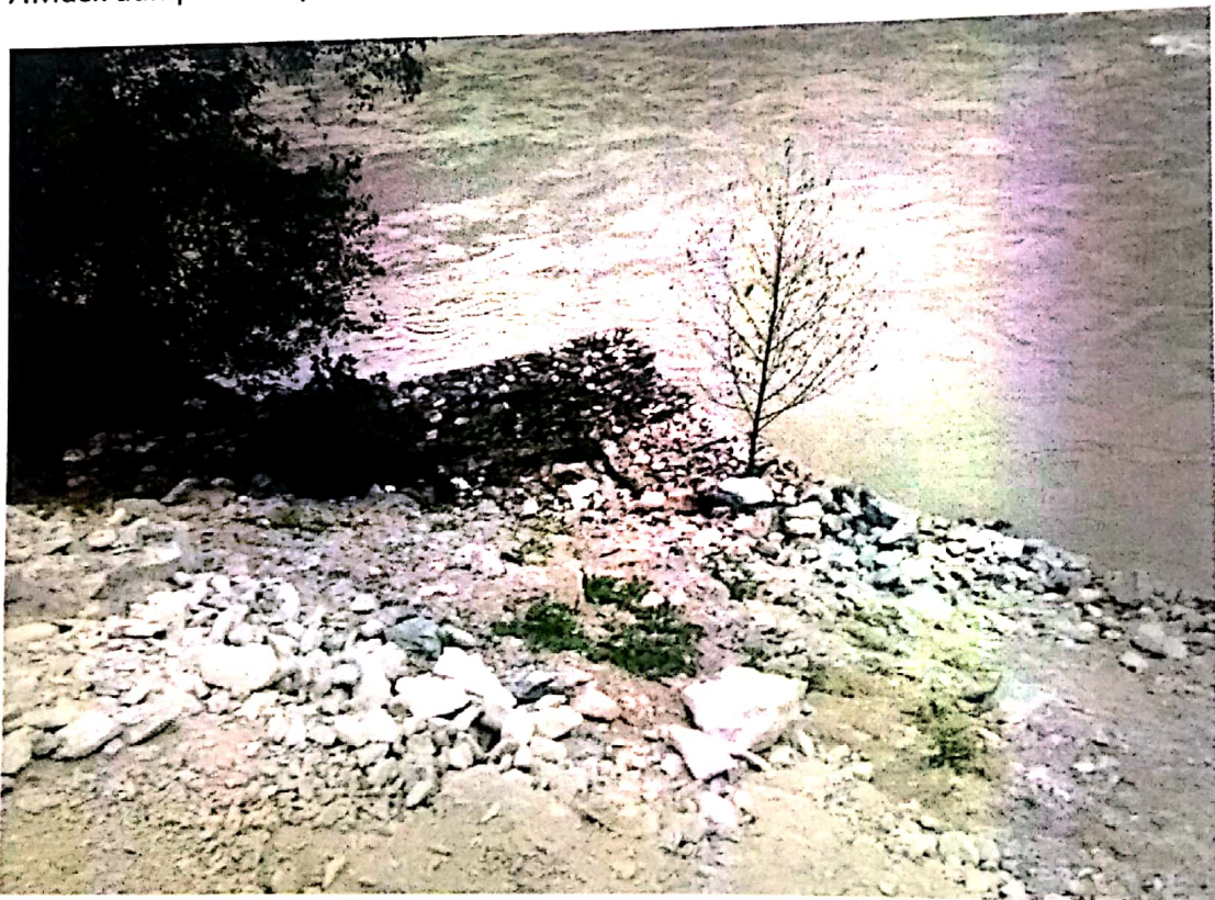
8. Muck dumped and protected towards river Beas: North End.
