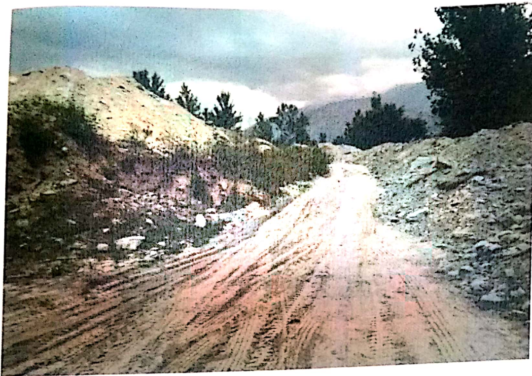
3. Muck dumped and protected, showing approach to the land.
